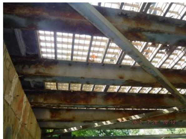
*Figure 2: Corrosion and Section Loss – Stringers*
