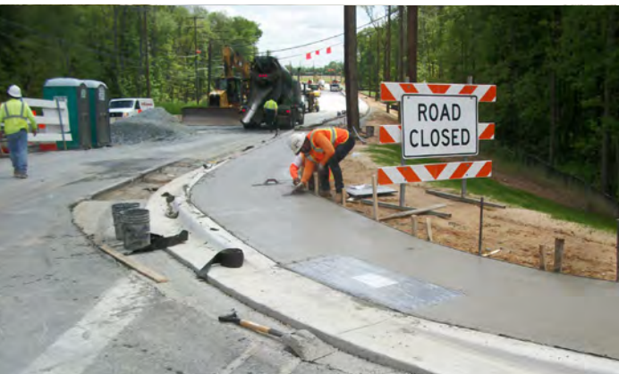
Roadway Improvements and Maintenance of Traffic
