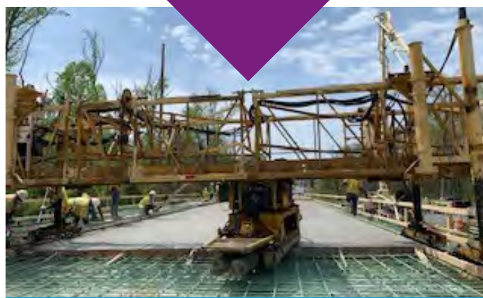
Bridge Repair, Reconstruction and Construction
