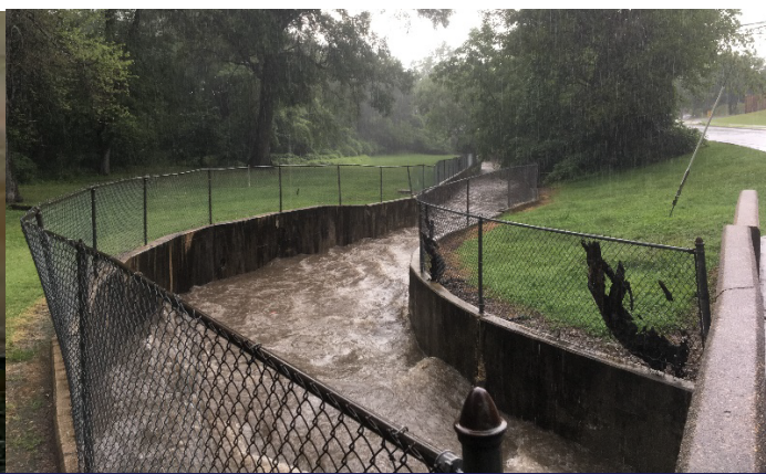
Storm Drain Improvement and Culvert Repair
