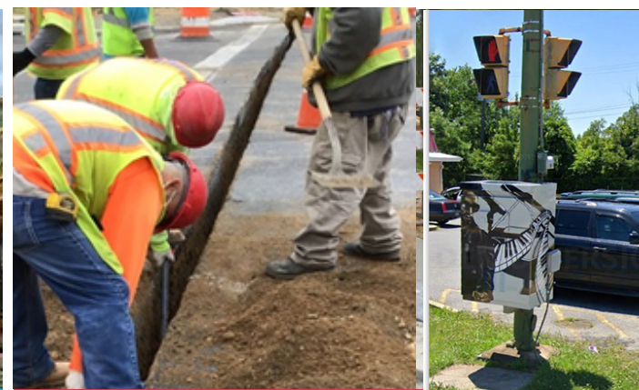
Intersection, Traffic Signal and Street Light Improvements
