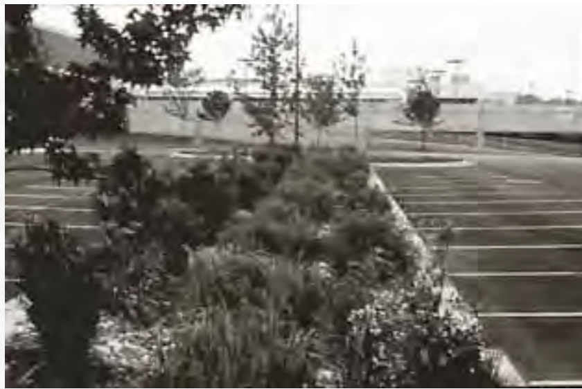
Figure 1-1. Parking lot bioretention area
