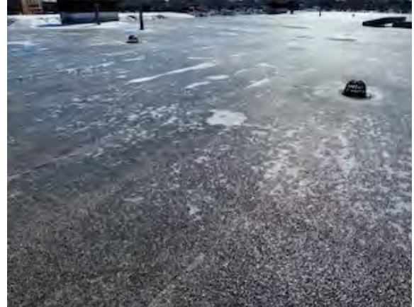
Photo #24: Flashing Caulk Roof Sample Set #27 – Non-ACM
