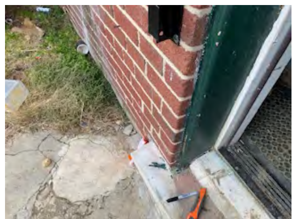
Photo #22: Exterior Door Caulk Sample Set #15 – Non-ACM
