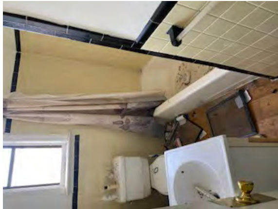
Photo #25: Typical Interior Window Caulk Sample Set #13 – Non-ACM
