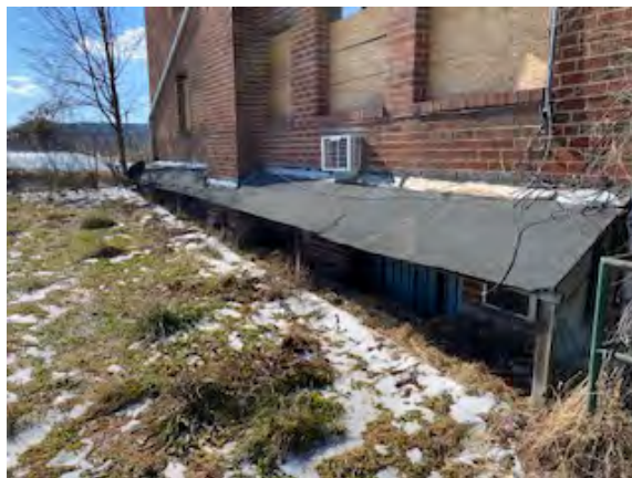
Photo #27: Asphalt Sheeting Small Rear Roof Sample Set #6 – Non-ACM
