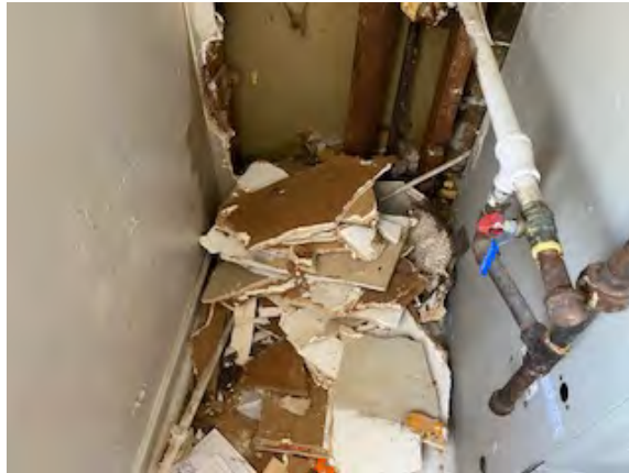
Photo #7: Typical Drywall Behind Plaster Wall Systems Sample Set #2 – Non-ACM
