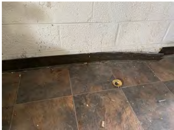
Photo #18: 4" Brown Covebase & Glue Laundry Room Sample Set #17 – Non-ACMs
