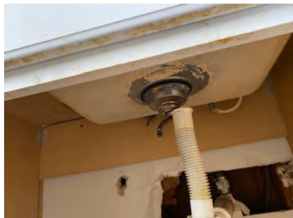
Photo #11: White Sink Undercoat/Insulation Unit 11 - Kitchen Sample Set #10 – Non-ACM
