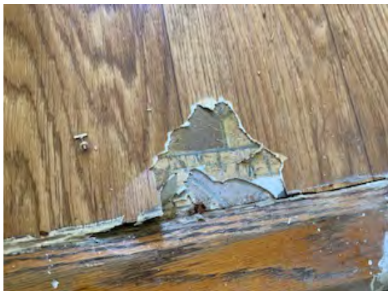
Photo #5: Typical 12" Colored Floor Tile & Glue Bathrooms Sample Set #21 – Non-ACMs
