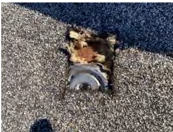
Photo #23: Rollled Asphalt Sheeting & Insulation Main Roof Sample Sets #7 & #8 – Non-ACMs
