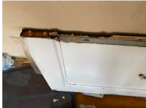
Photo #14: Cross Cut of Typical Fire Door No Suspected ACM
