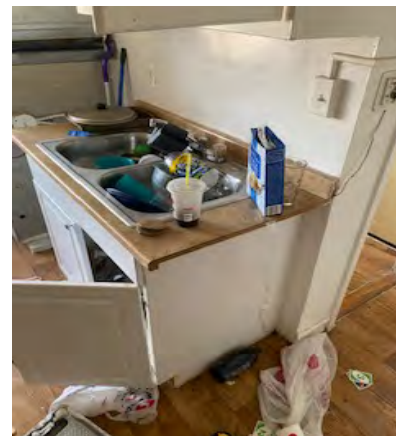
Photo #4: Typical Counter Caulk Kitchens Sample Set #14 – Non-ACM
