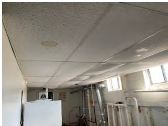
Photo #16: 2'x4' Pinhole Ceiling Tile Laundry Room Sample Set #5 – Non-ACM
