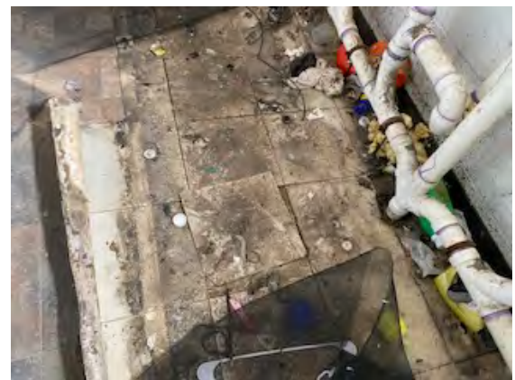
Photo #17: 12" Brown Pattern Linoleum & 12" White Floor Tile & Glues – Laundry Room Sample Sets #18 & #19 – Non-ACMs
