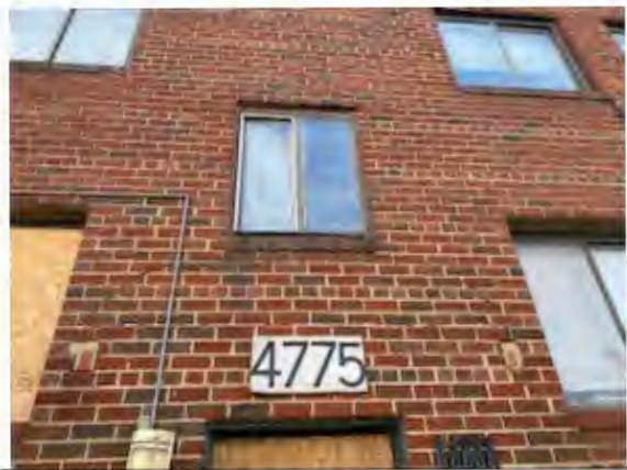
Photo #2: Site Address
