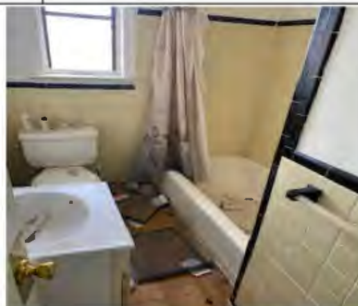
Photo #10: Typical Bathroom Components Note – Ceramic Components are the Same as ones tested in 4785 – No Elevated Lead
