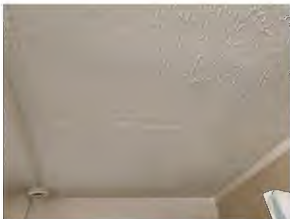
Photo #7: Typical Ceiling Components No LBP
