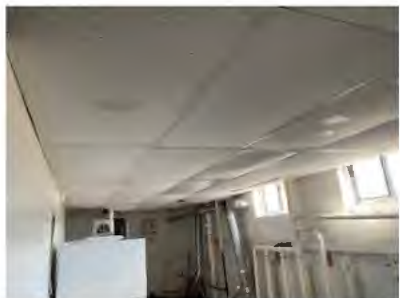
Photo #9: Laundry Room Components No LBP
