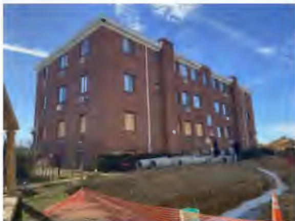
Photo #1: Front of Site
