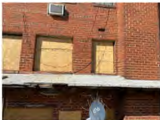
Photo #19: Asphalt Roof Shingles & Paper Rear Small Roof Sample Sets #6& #7 – Non-ACMs
