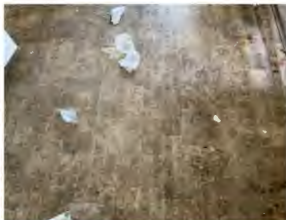
Photo #20: Rectangle Stone Pattern Linoleum & Mastic Unit 9 Sample Set #18 – Non-ACMs
