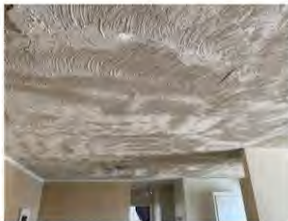
Photo #14: Thick Textured Ceiling Unit Ceilings Sample Set 2 – Non-ACM
