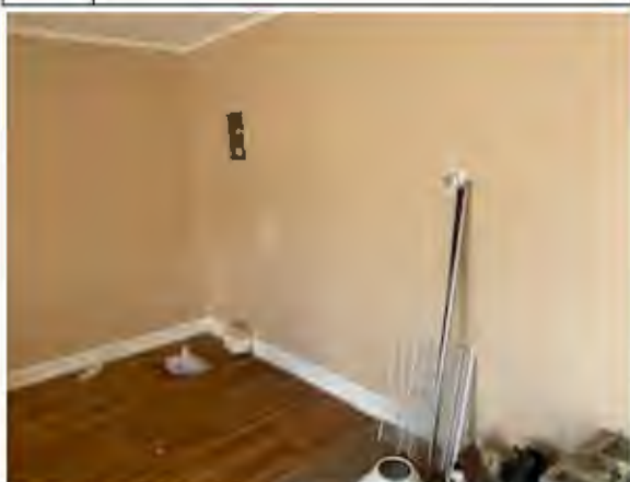
Photo #3: Typical Plaster Walls – 2 Layers Throughout Building Sample Set #1 – Non-ACMs
