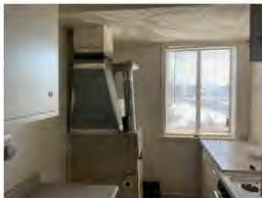
Photo #16: Typical Counter Caulk Kitchens Sample Set #9 – Non-ACM
