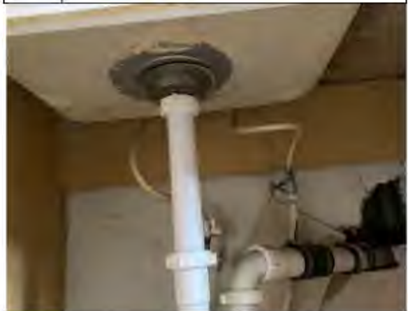
Photo #12: White Sink Undercoat/Insulation Sporadic Locations Sample Set #15 – Non-ACM
