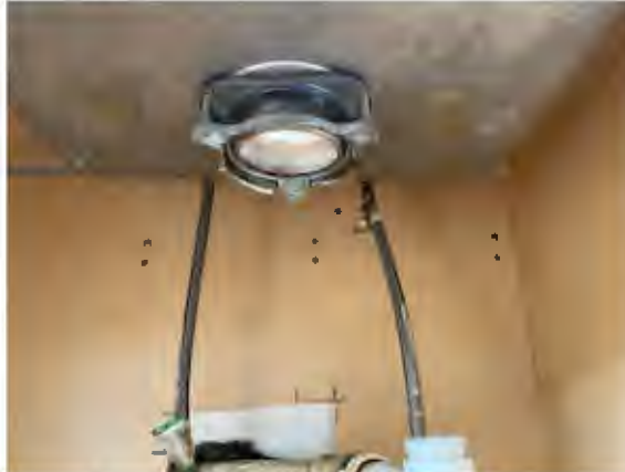
Photo #6: Typical Unit No Sink Undercoating/Insulation
