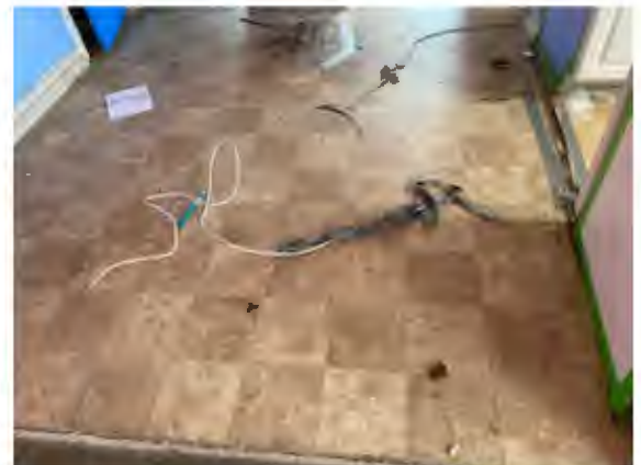
Photo #10: 9" Beige Stone Pattern Linoleum & Mastic Unit 12 Sample Set #16 – Non-ACMs
