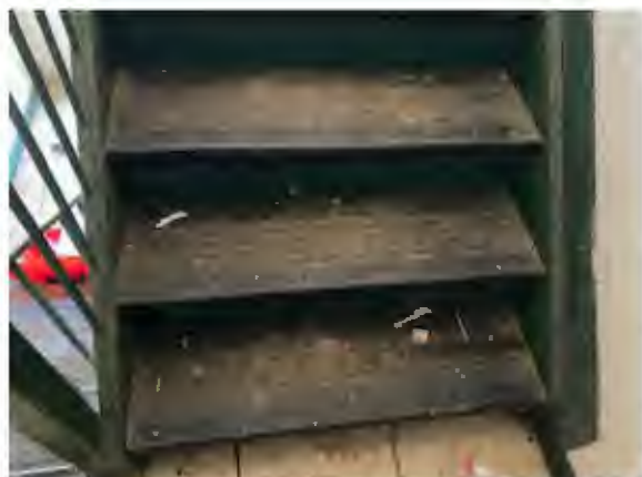
Photo #21: Vinyl Stair Tread and Glue Hallway Stairs Sample Set #14 – Non-ACMs
