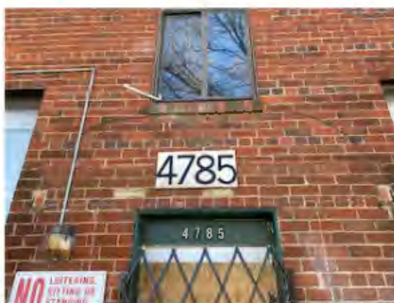
Photo #2: Site Address
