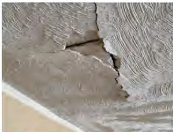
Photo #13: Thick Textured Ceiling Unit Ceilings Sample Set 2 – Non-ACM
