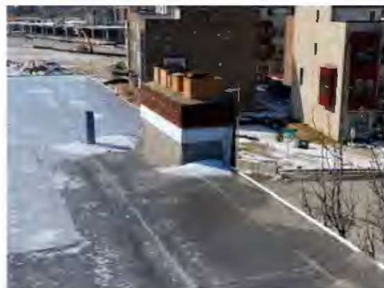
Photo #22: Roof Flashing Caulk Main Roof Sample Set #5 Non-ACM
