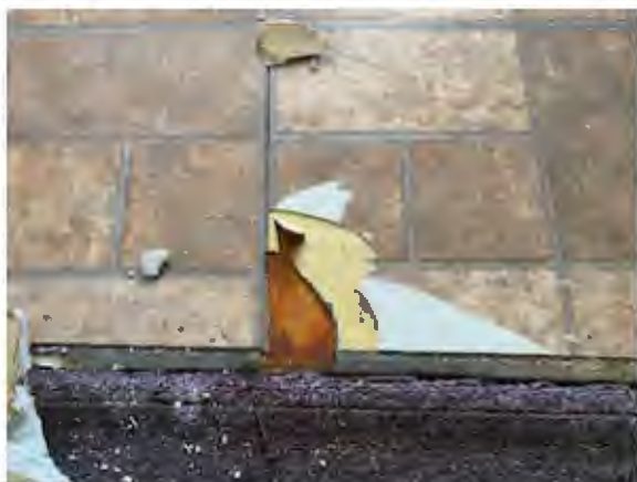
Photo #17: 12" Brick Pattern Floor Tile, 12x12 White Floor Tile & Mastics – Unit 10 Kitchen Sample Sets #19 & 20 – Non-ACMs
