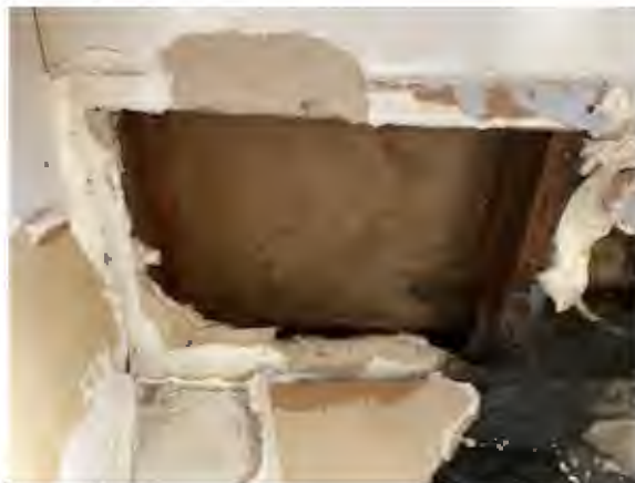
Photo #18: Typical Drywall Behind Plaster Throughout Building Sample Set #4 – Non-ACM
