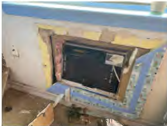
Photo #9: Typical Drywall Behind Plaster Throughout Building Sample Set #4 – Non-ACMs
