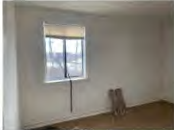
Photo #4: Typical Bedroom Components No LBP
