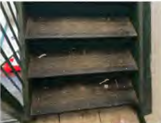
Photo #5: Stair Components No LBP
