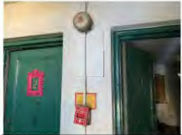
Photo #8: Typical Hallway Components No LBP
